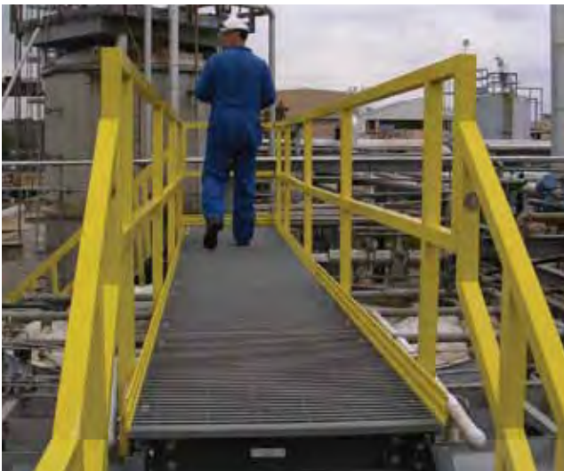
SAFRAIL™ and DURAGRID® pultruded grating were fabricated to make access platforms over waste water recycling tanks. The previous steel structure corroded, and was unsafe.
