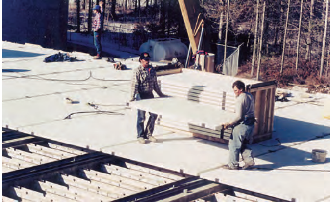
DURASHIELD® panels are used as plant roofs and chemical tank covers in corrosive environments, such as the covers (16,800 s.f.)(1,560 m 2 ) over anaerobic digester units pictured above.
