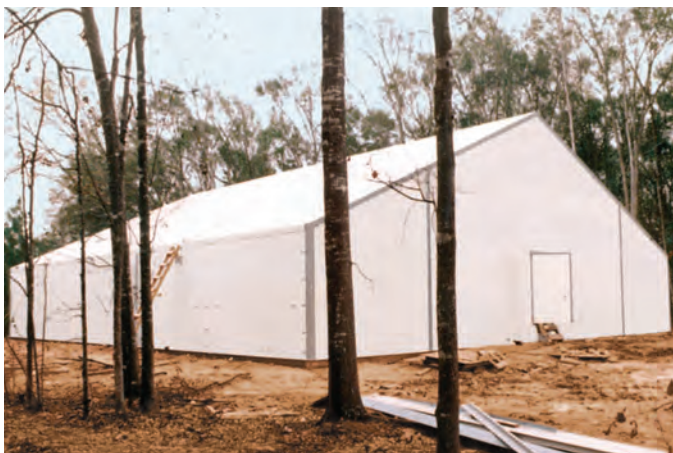
Compaq Computer chose a foam core panel building to assure RFI/EMI compliance for attenuation.
