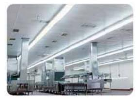
**Redco™ FRP** textured wall panels are ideal for food processing plants, hospitals, restaurants, even car washes. FRP sheet is easy to clean and keeps drywall from getting wet and damaged, preventing any mold or fungus growth in wet environments.
